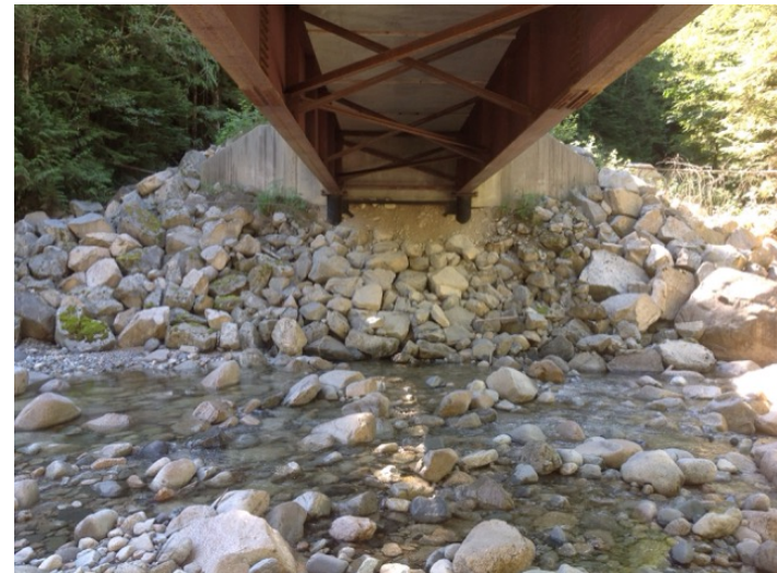
Left Bank Abutment when facing downstream
