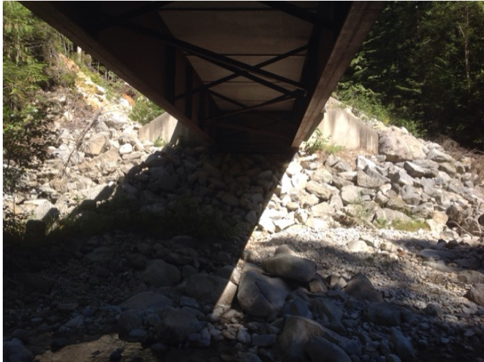
Right Bank Abutment when facing downstream
